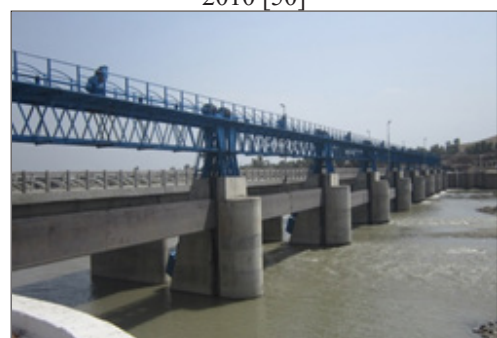
Figure 25: Munda Headworks in 2016 after restoration/ Reconstruction [50]
