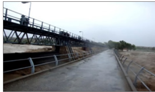
Figure 23: Munda Headworks during flood 2010 – flow above the structure [50]
