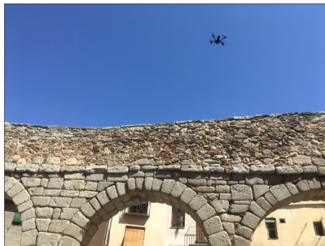
Figure 1: Quadrotor drone flying over the Roman Aqueduct of Segovia, for inspection (photo by the author).
