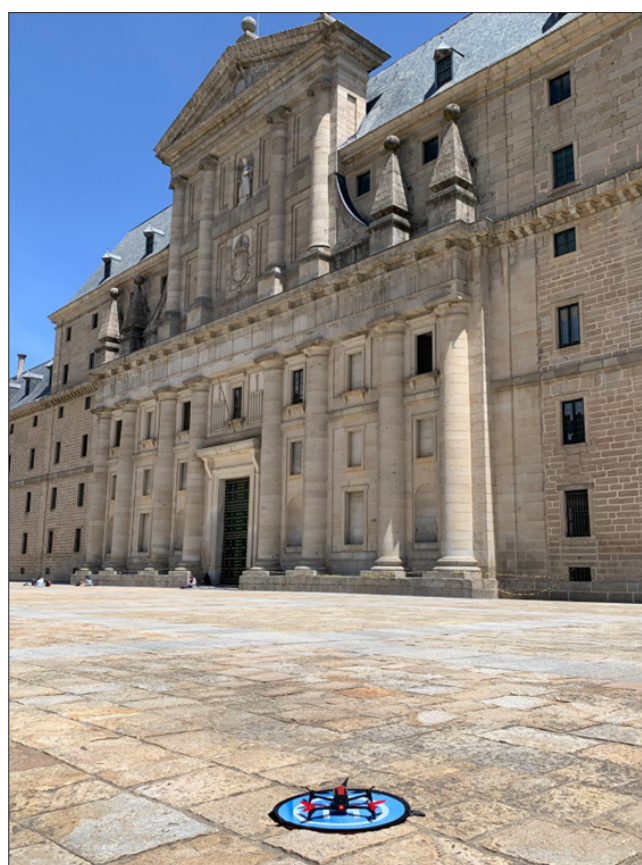
Figure 2: Quadrotor drone ready to take off, for an inspection on the main facade of the Monastery of El Escorial, Spain (photo by the author).
