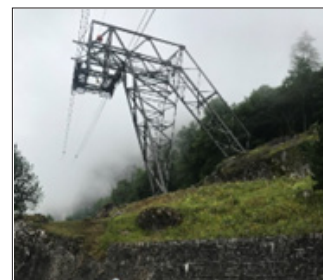
Figure 3: Cableway placed in altitude. Metallic structure supported by concrete basements.
