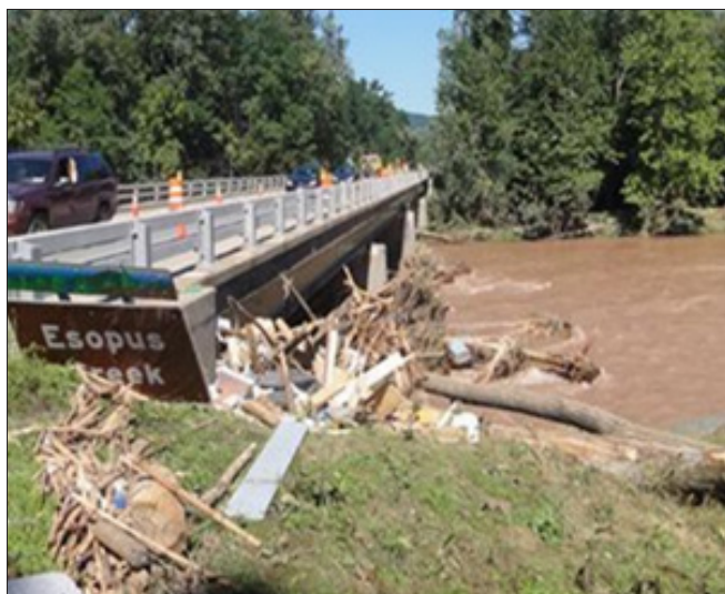
Figure 1a: Woody debris blocked by a bridge (McDonald et al., 2004)
