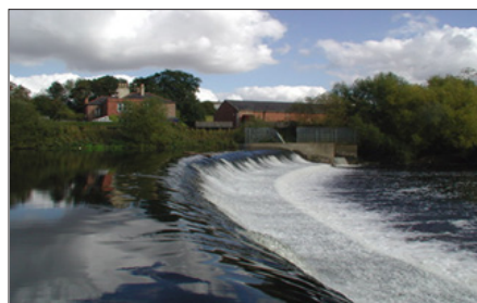
Figure 3d: River Wharfe Weir at Tadcaster (Glazzard, 2007)
