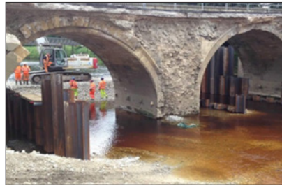
Figure 3f: Sheet piled wall in Tadcaster (Aeyates, 2018)
