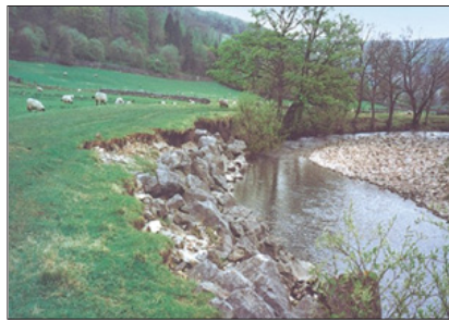
Figure 11a: Blackstone Bank Revetment to avoid erosion due to gravel deposition (Environment Agency, 1999)
