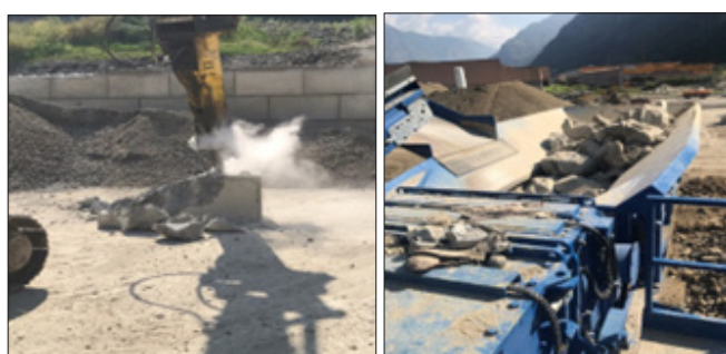
Figure 1: Demolition and crushing procedure of the concrete produced with natural aggregates.
