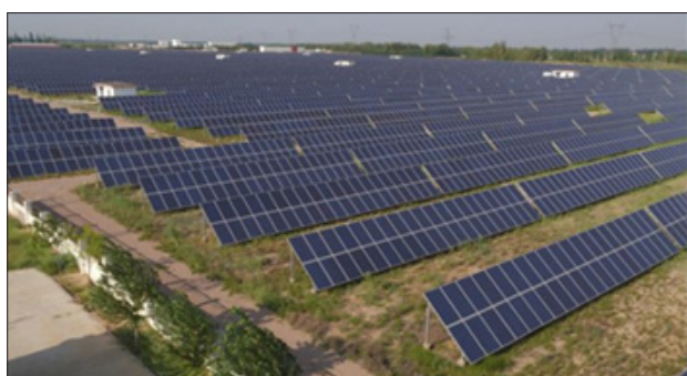
Figure 3: Solar panels reduce near-surface wind speed, temperature and soil evaporation to facilitate the growth of soil and water conservation vegetation (Dengkou, China) restore vegetation in order to make the goods and services vegetation ecosystem give to meet the needs of human production and life.
