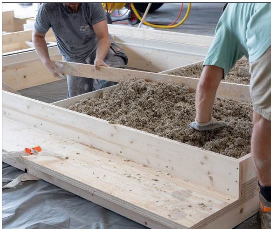
(a) Filling timber frames with hempcrete
