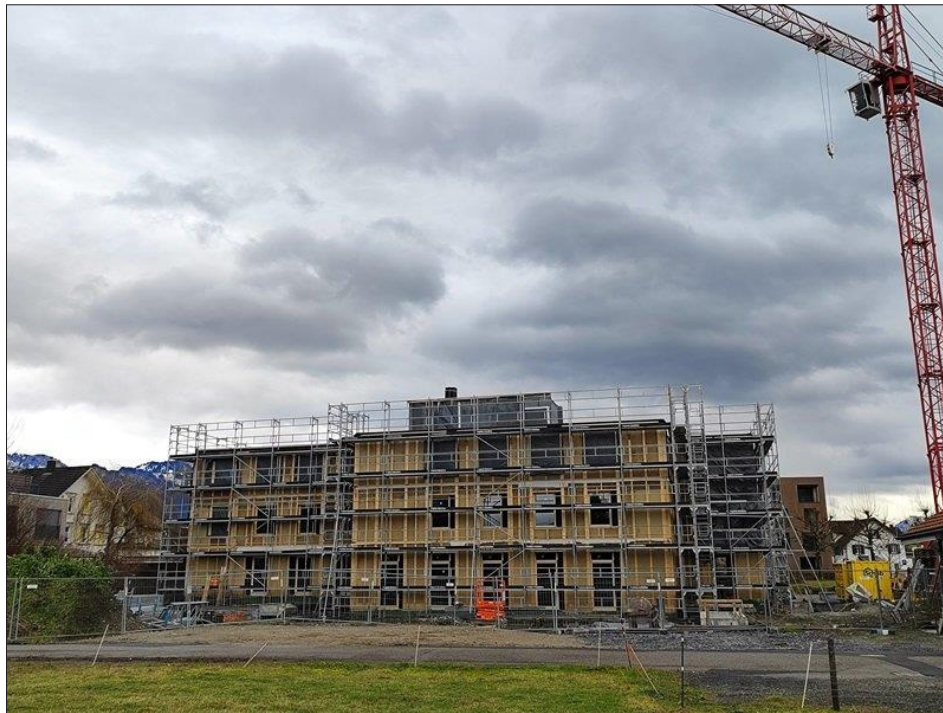
(a) Construction Progress
