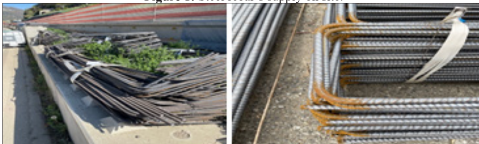
Figure 1: Steel rebar's supply on site.
