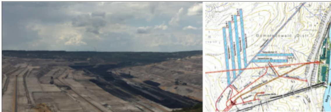
Figure 4: Pumped hydro storage power plant in open-cast mines – example Hambach open-cast mine (left image), example pipe caverns (right image) (Schmidt-Böcking et al., 2013), (Schmidt-Böcking et al., 2023).
