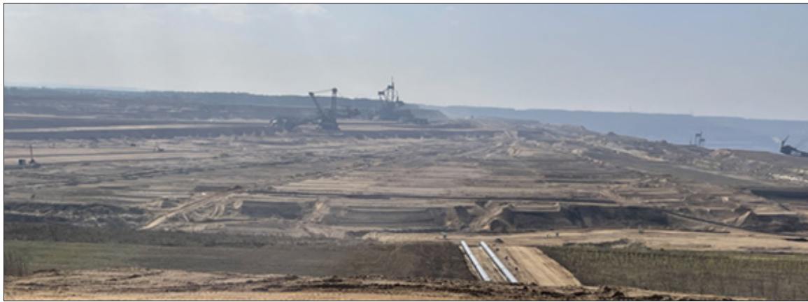
Figure 6: View of the Manheim Basin (Manheimer Bucht) – in the current excavated area, potential location of the upper reservoir (own photo)
